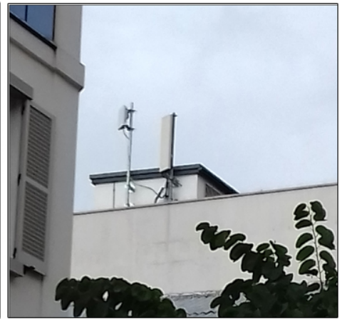
5G antennae at the Courthouse.
